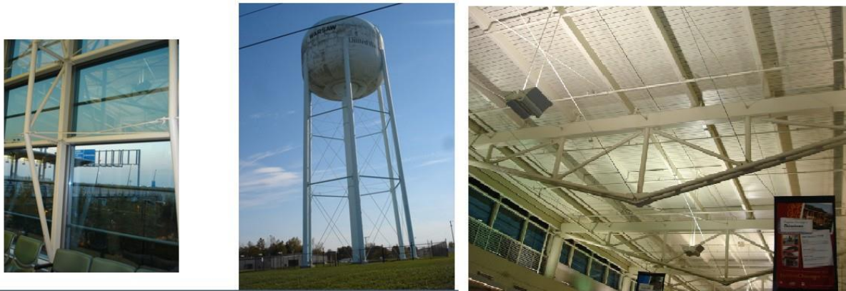
Tie Rods in Structures
